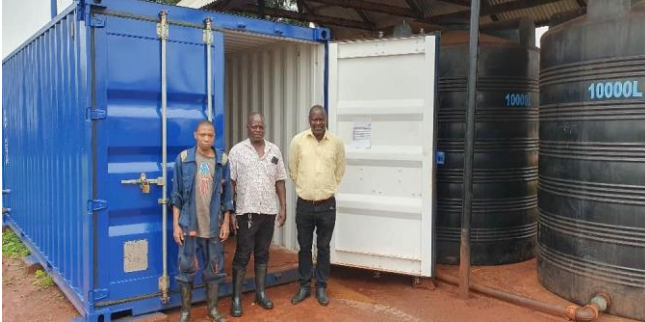
Water filtration renovation at Kwaraguru estate
