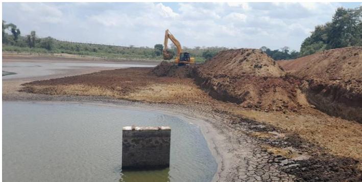
Deepening and widening of Kwaraguru dam
